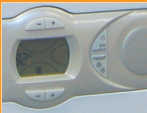
LCD diagnostic boiler fascia panel
