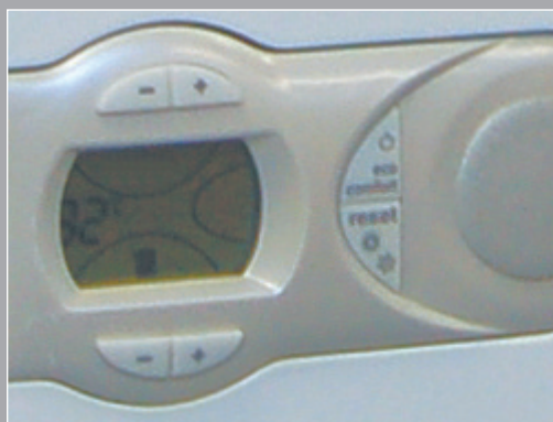
LCD diagnostic boiler fascia panel
